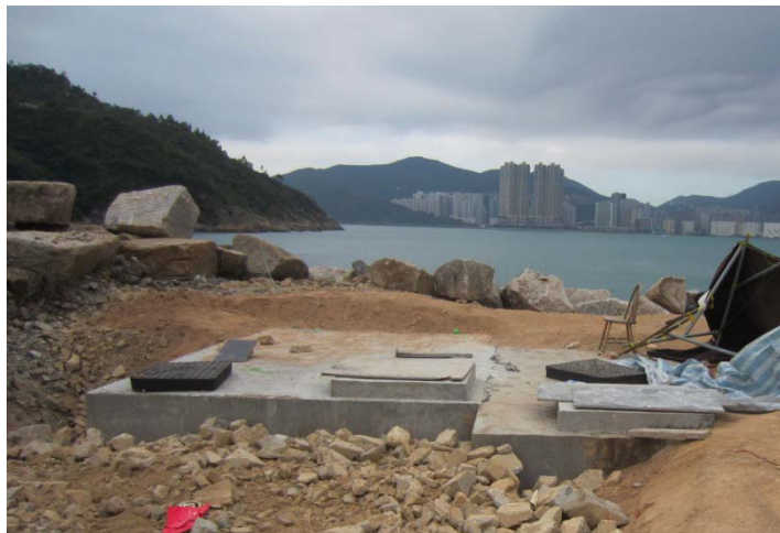
Photo 2 – Construction of the new beach manhole has been largely finished, with only small part of backfilling and reinstatement works remaining.
