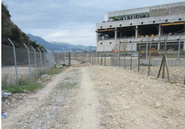
Photo 1 – Construction of the land duct has been finished and the site has been reinstated to its original conditions.
