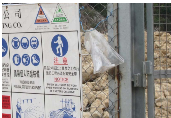
Photo 3 –The EP copy displayed at the vehicular site entrance was damaged.
